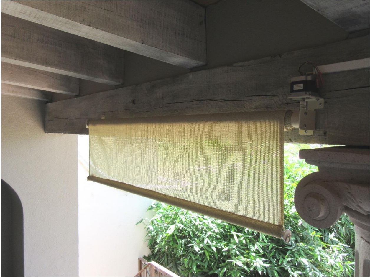
Figure 9 - Installed Shade with Motor Drive
