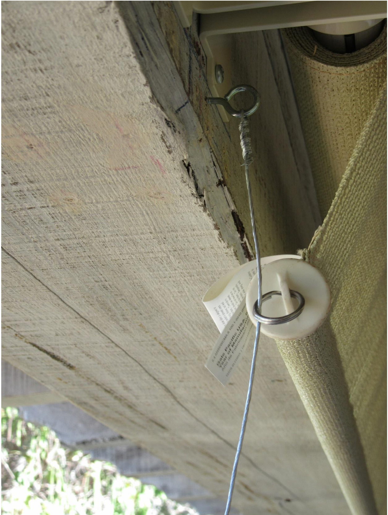
Figure 21 - Using Wire Guides on Shades
