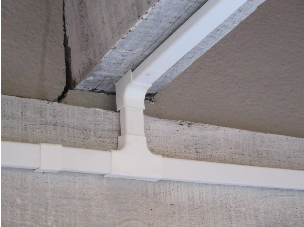
Figure 10 - Channel for Routing Motor Cables
