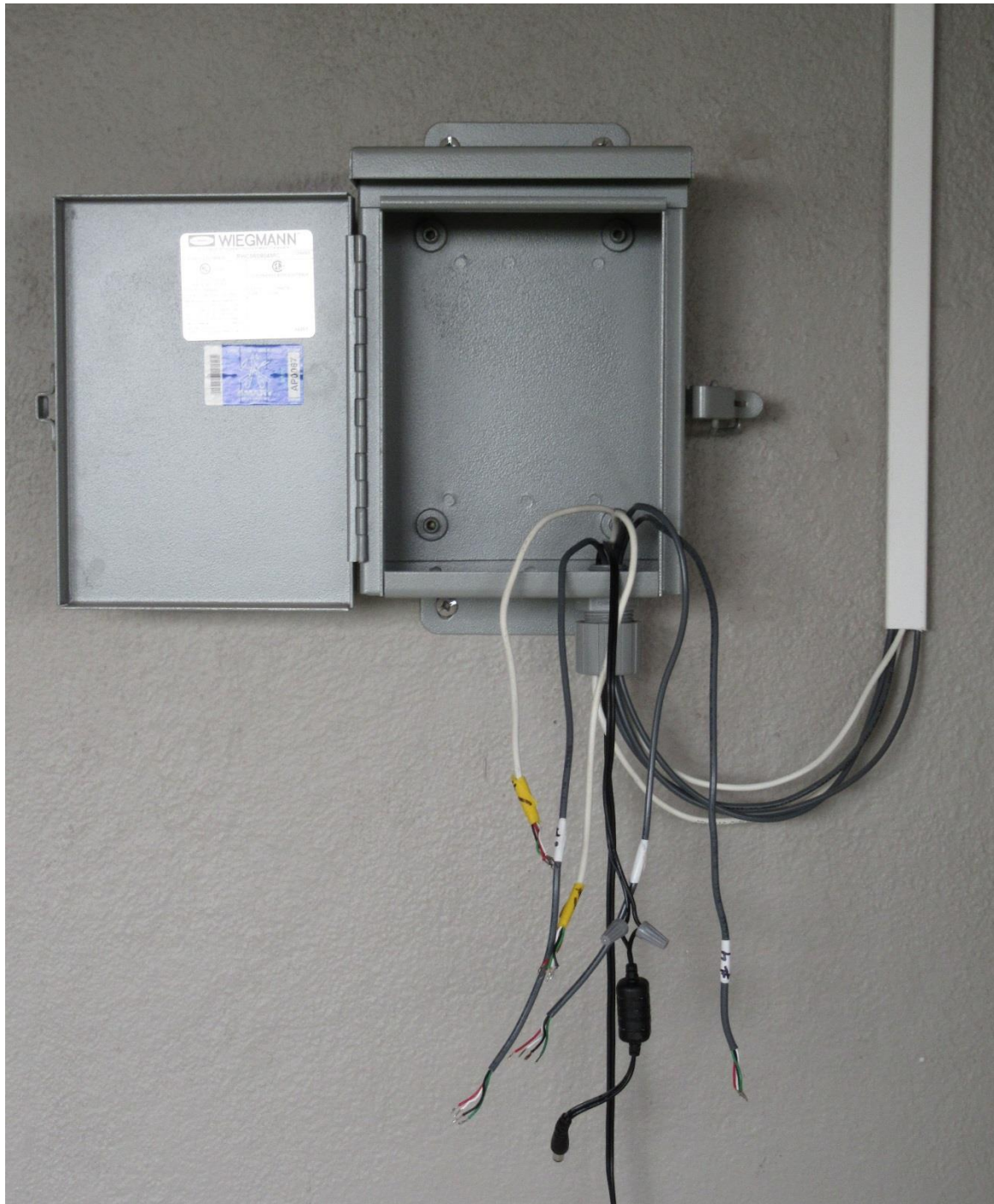
Figure 13 - Control Panel Box with Wires Routed through Cable Clamp
